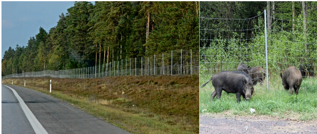
Figure 1. Left: Traditional moose exclusion fences in southern Sweden combined with a fine-meshed lower fence to prevent accidents with wild boar. Photo: Andreas Seiler. Right: Wild boar family benefitting from a hole in a fence. Photo: Mattias Olsson.
