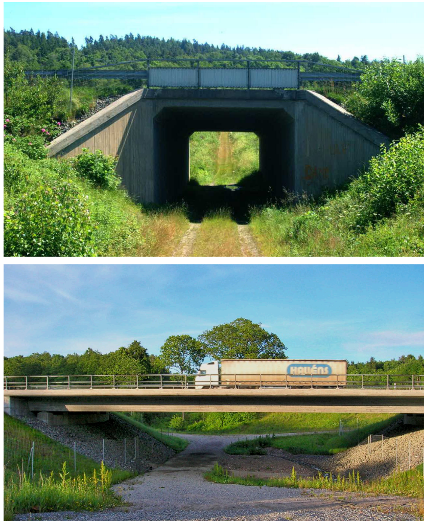
Figure 8. Conventional bridges over a private forestry road (above) and in combination with an extended wildlife passage (below). Both bridges provide a potential passage to wildlife and have been monitored using sand beds (Seiler and Olsson, 2009). Due to its small size, the upper passage is significantly less effective in providing connectivity to wildlife than the larger passage below. Yet, it may nevertheless be sufficient to support the movements of those individuals that otherwise might attempt to breach the fence along the road and impose a traffic hazard. Thus, even the smaller bridge may be fully efficient in reducing WVC. Photos: Andreas Seiler.
