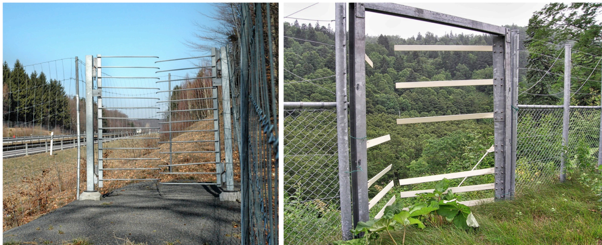
Figure 4. Left: experimental one-way gate for moose and roe deer in Sweden (Photo: Mats Lindquist). Right: experimental one-way gate for sika deer in Hokkaido, Japan (Photo: Andreas Seiler). Efficacy of both gate types is unknown. Due to the risk of failure, one-way gates are no longer recommended.
