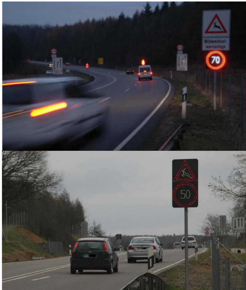
Figure 7. Crosswalk with an animal detection system and a deer warning unit in Aglasterhausen, Germany. Source: Strein et al. (2008).
