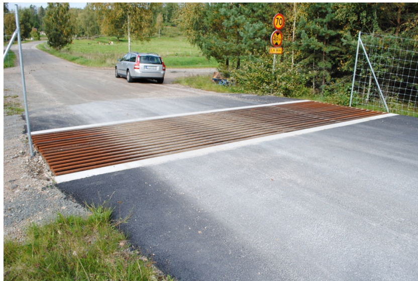
Figure 5. Cattle/wildlife grid over a private road connecting with a highway near Osby, southern Sweden. Efficacy in preventing moose or deer from entering the road is unknown. Photo: Mattias Olsson.
