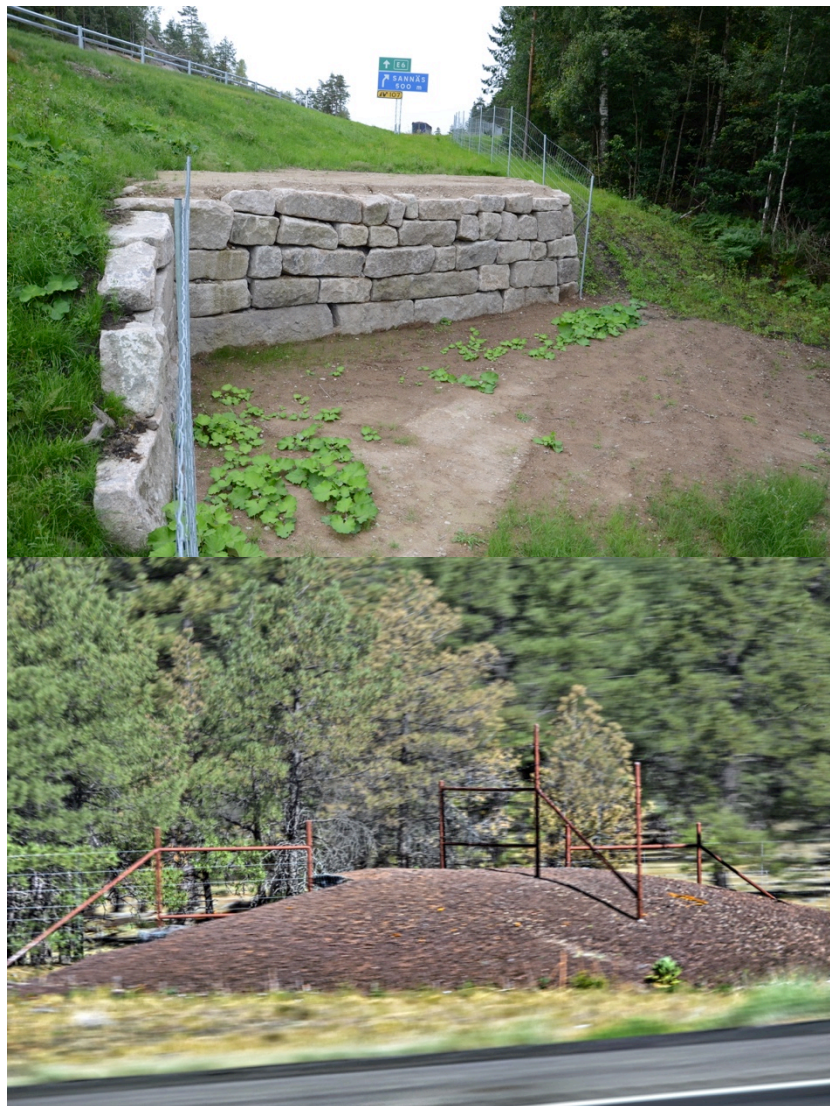
Figure 3. Upper picture: jump-out in southern Sweden (Photo: Mattias Olsson). Lower picture: escape ramp seen from the roadside in Arizona, USA (Photo: Andreas Seiler).
